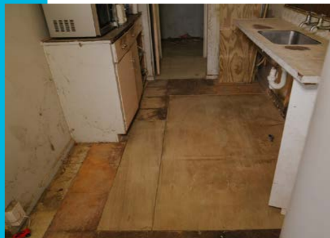
Replacing the rotting floorboards in the kitchen.
