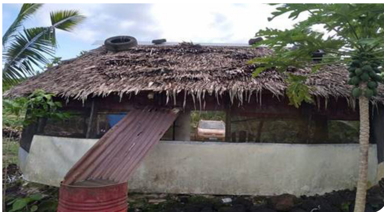
Figure 6: Makeshift rainwater harvesting system
