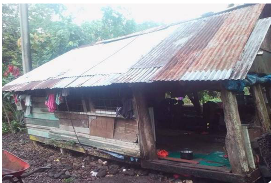
Figure 4: Unsafe shelter in urban Apia with VIP latrine
