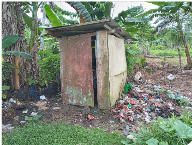
Figure 7: (right) Rural household with VIP latrine
