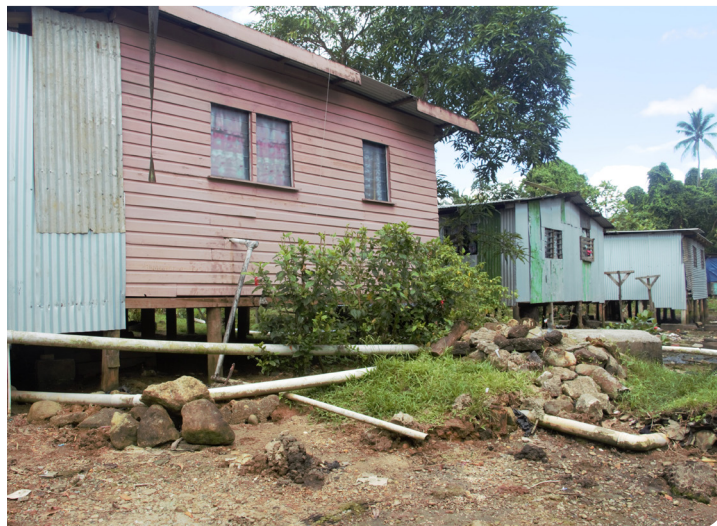
Figure 14 - Outlet for septic tanks at an informal settlement in the Lami area being directed into the mangrove area it is situated next to.
