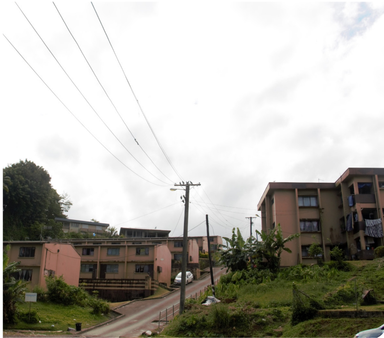
Figure 9 - A Public Rental Board Estate in the Raiwai area. One flat in the triple storey building on the right houses a single mother with 6 children, in an open plan 23m 2 unit, with no bedrooms for privacy.
