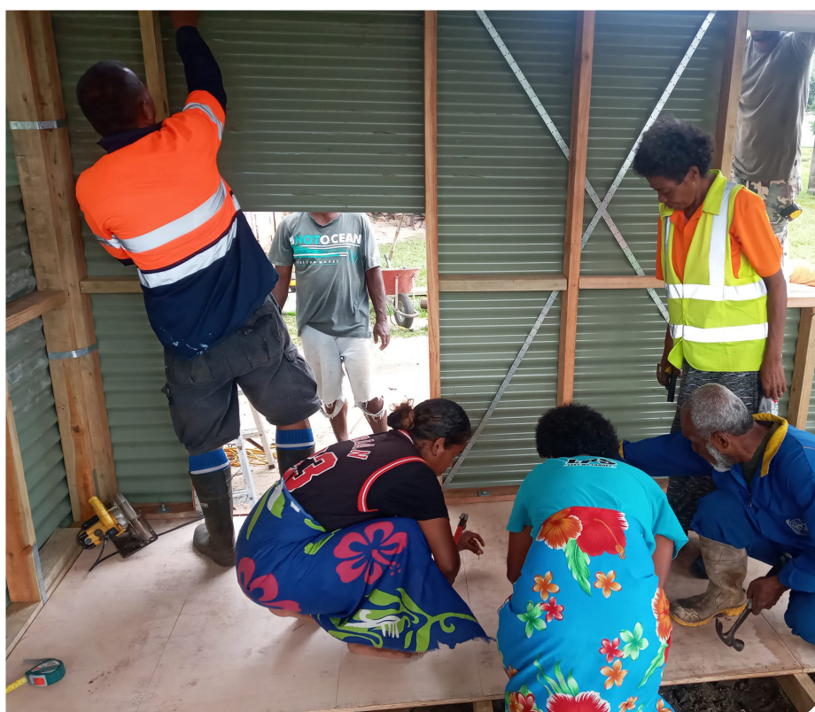
Figure 6 – Men and women participating in a Build Back Safer Training in a Village in the Lomaiviti Province
